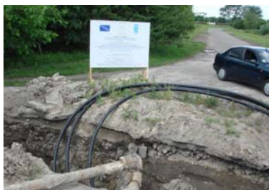
Repair of water supply system, Yerkivtsi village of Kyivska oblast
