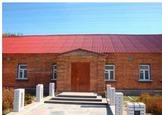
New roof of local health post, Vysoke village, Zhytomyrska oblast
