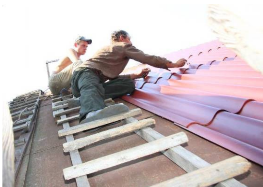
Implementing community project on energy saving (roof replacement)
