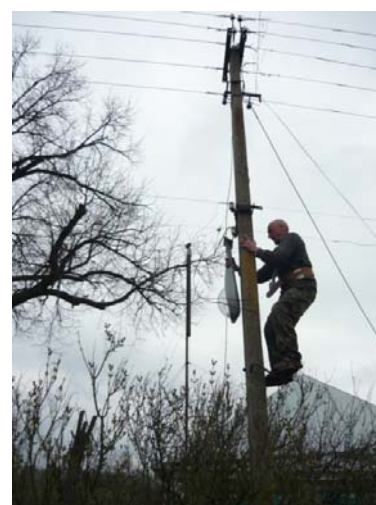
Energy saving light-bulbs are installed in Or dovka village, Kharkivska oblast
